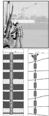
Installation in fractured bedrock
