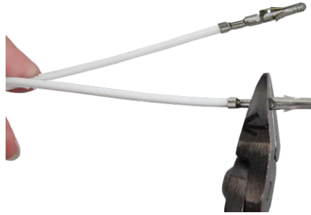
Cut the Pins on Each Tape/Cable Lead in Half (as shown)
