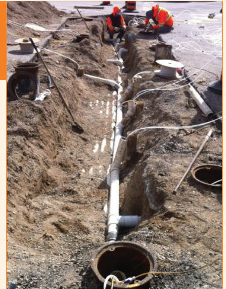
Waterloo Emitters were installed as a fence to cut-off migration of a contaminant plume.
